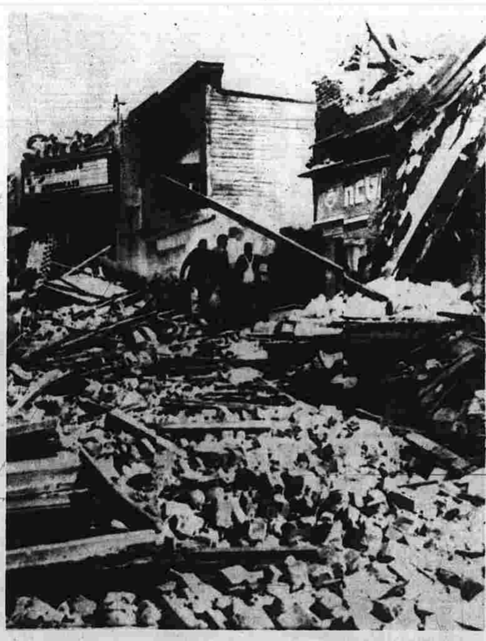
Rubble lies in streets of Port Jervis, N. Y. Friday after building collapsed.
